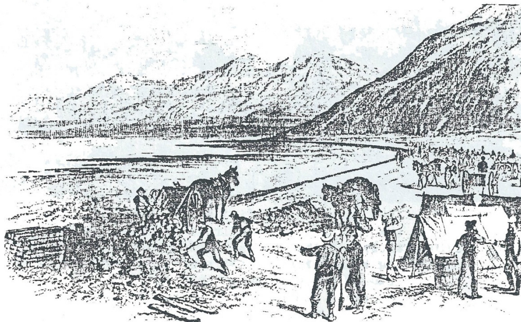
Mormon volunteer laborers helping construct an extension of the transcontinental railroad from Ogden to Salt Lake City in 1870.
